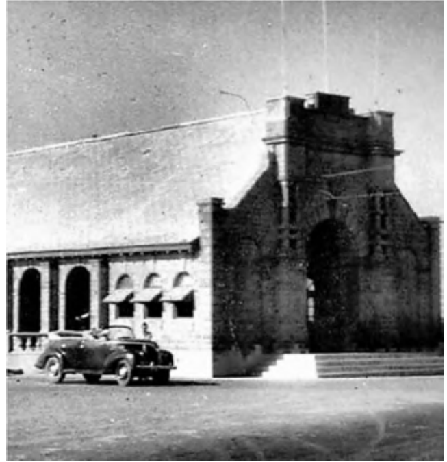
Figure 2: Prince of Wales pier © Khaled Mashaba
